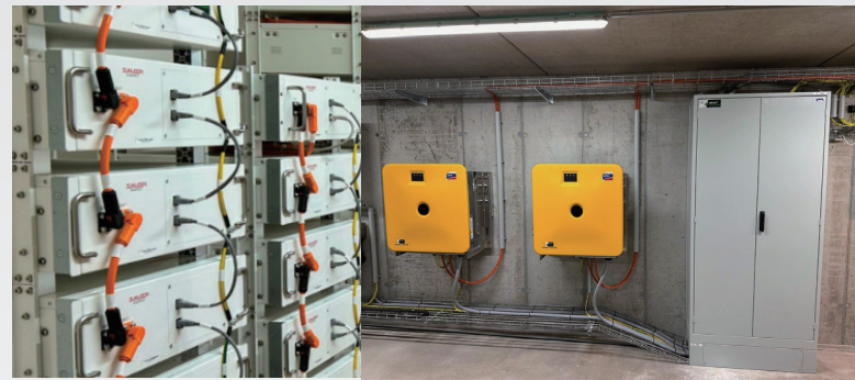
Austria OASIS Flex & SMA 100kW/480kWh Rack-mounted Battery System BESS for Commercial Building
