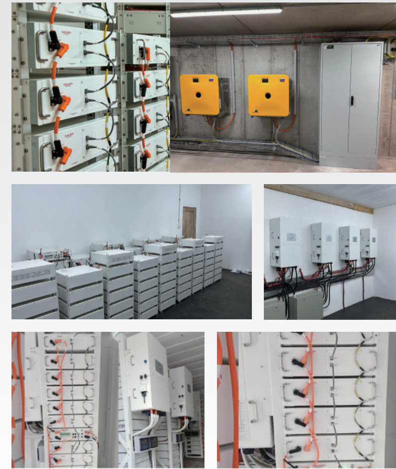
Austria OASIS Flex & SMA 100kW/480kWh Rack-mounted Battery System BESS for Commercial Building
