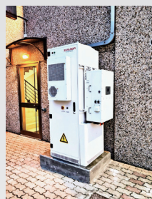
Italy OASIS 60 50kW/60kWh Outdoor Battery Cabinet System
