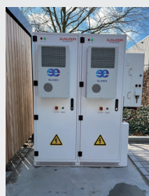
Holland OASIS 60 50kW/120kWh Outdoor Battery Cabinet System
