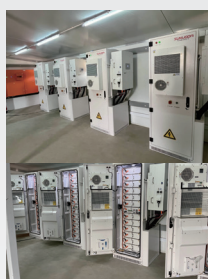
South Africa OASIS 60 & Deye 200kW/240 kWh Outdoor Battery Cabinet System
